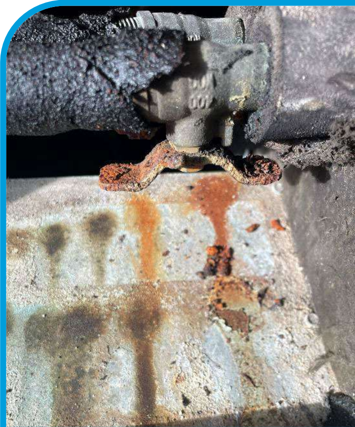
Valve corrosion
