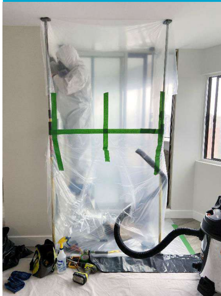
2. Fan coil removal
