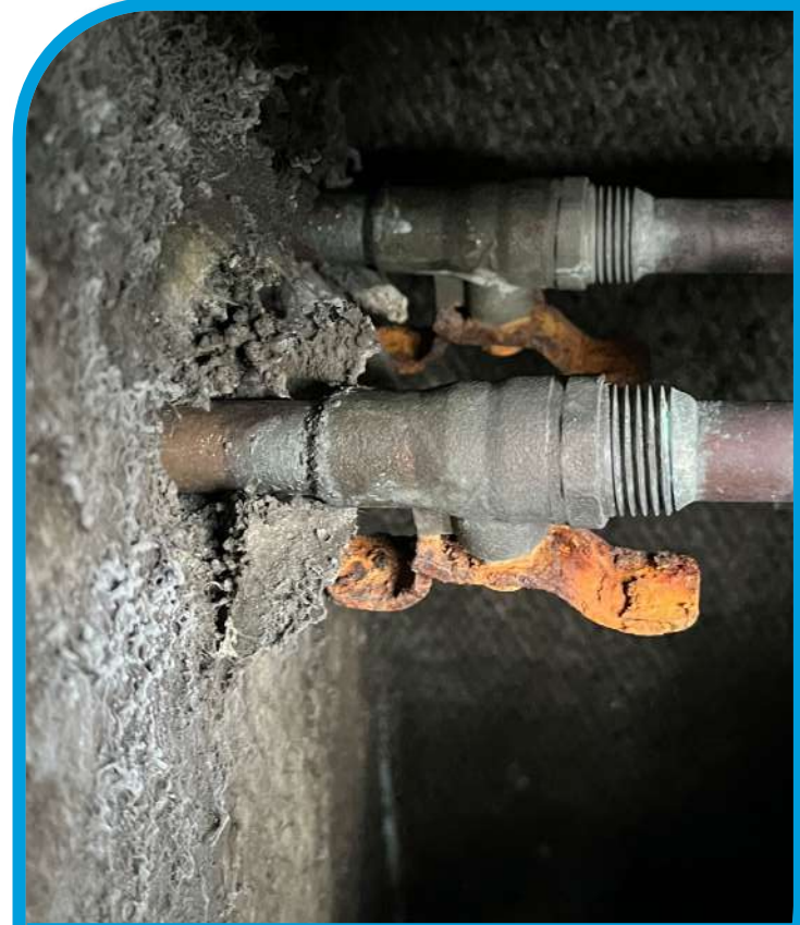
Valve corrosion
