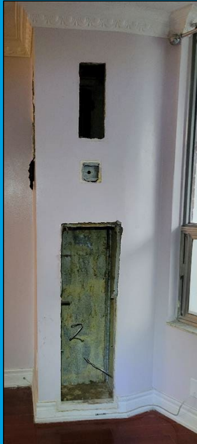
2. Wall cut to standard height. Old Insulation removed
