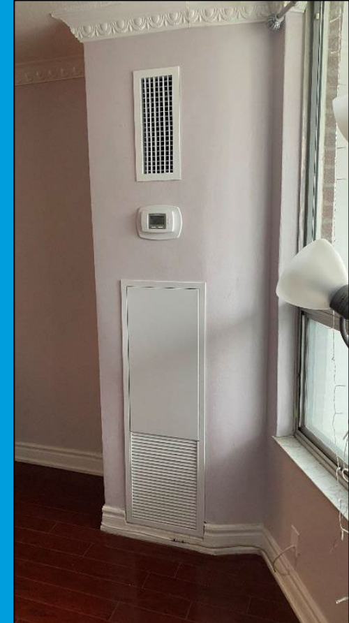
4. New FCU, Thermostat and Door Installed
