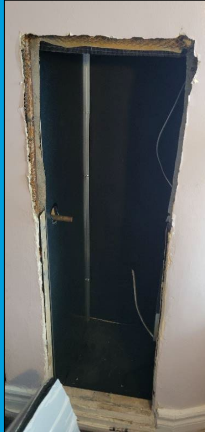
3. Cabinet cleaned and reinsulated
