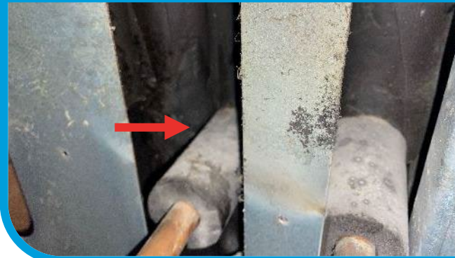
Insulation peeled back
