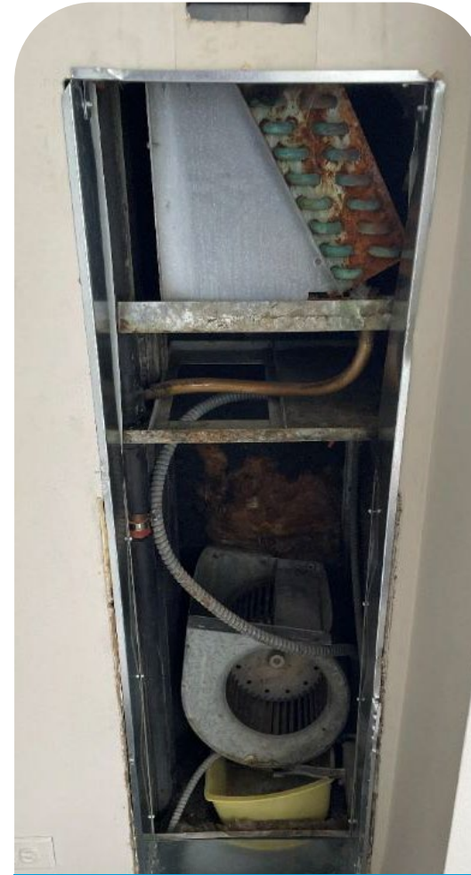
Metal Trim Installed
