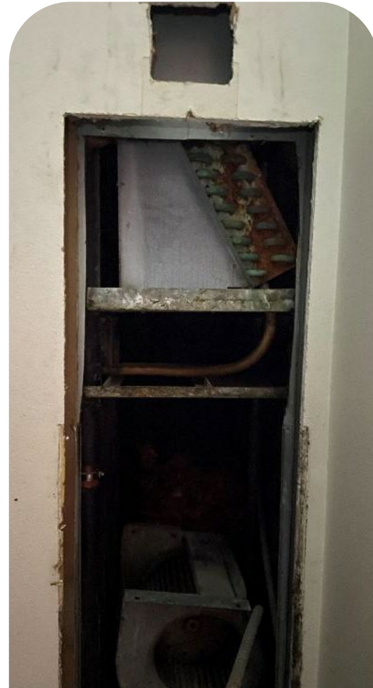
Wall cut to 4'
