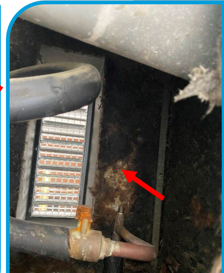
Upper Cabinet Wall
