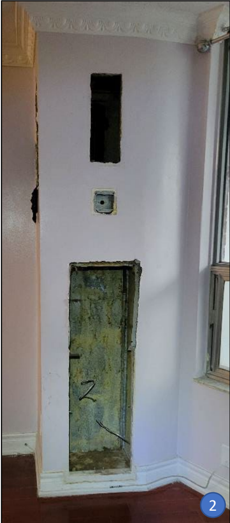
Wall cut to standard height and old insulation removed
