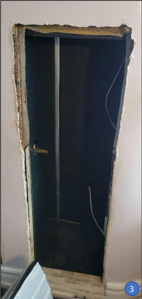
Cabinet cleaned and re-insulated
