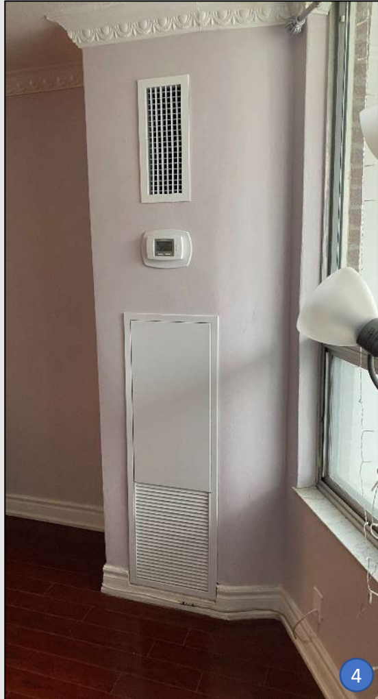
New fan coil installed complete with new access door
